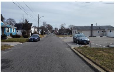
roadway features were found to be in excess of 400 feet in each direction. These values are greater than the 155-foot minimum stopping sight distance required according to AASTHO criteria for the speed limit, and the 205 feet for the observed travel speeds between 20 and 30 mph observed along the local roads.
